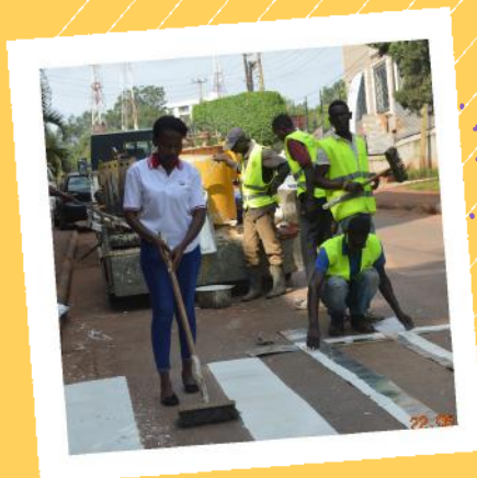
Road safety campaign, Zebra Crossing at Ssezibwa road in 2021
