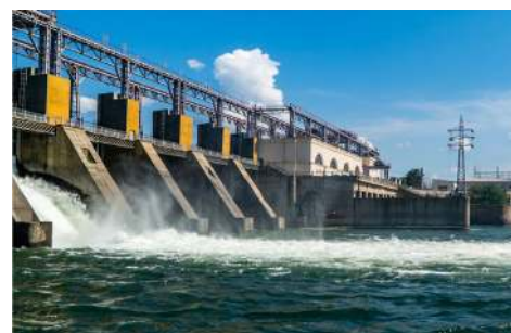
Bujagali Power Plant
